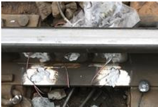
Field test (discontinuous)
